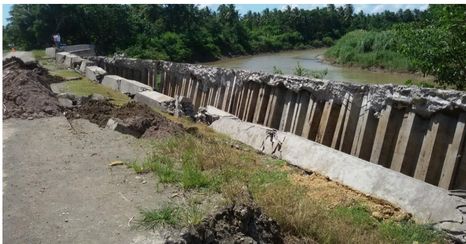
Figure 4. Flood Control Building
