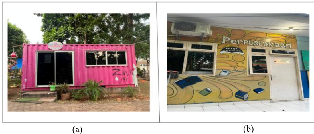
Figure 8. (a) locked container library, (b) locked reading room
