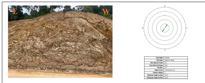
Gambar 6. Fault Litologi Dasit Area Akses Magazine
