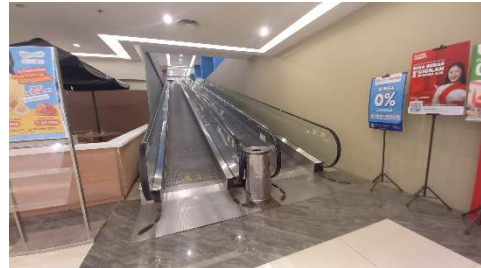
Gambar 20. Ramp Berjalan di Manado Town Square. Sumber: Peneliti, 2025
