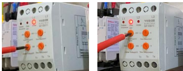
Gambar 12. Setting Time Phase Failure Relay
